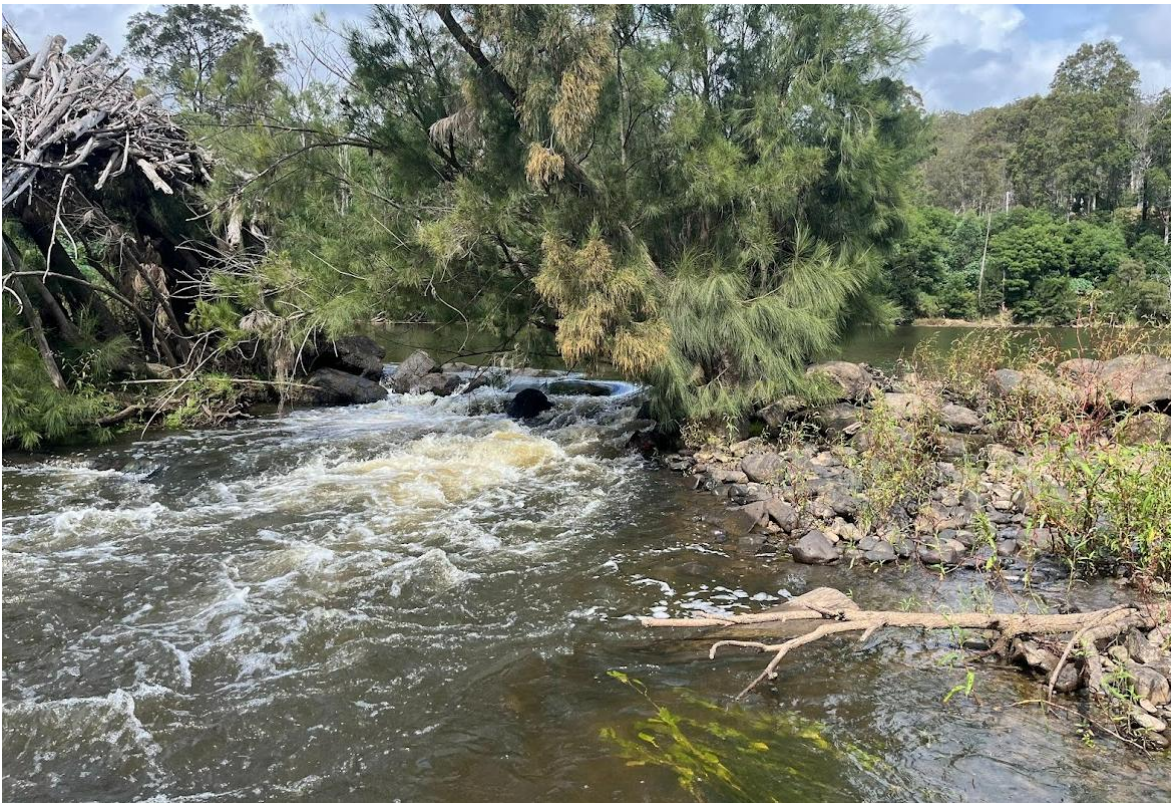
Photo 2: One breach of the weir (photo taken downstream of the weir)
