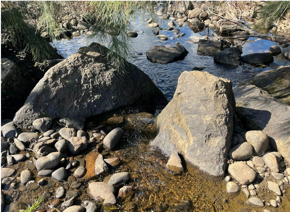
Photo 11: Example of existing weir exhibiting 1:20 grade and avoiding vertical drops greater than 100mm in height and concentrated areas of velocity
