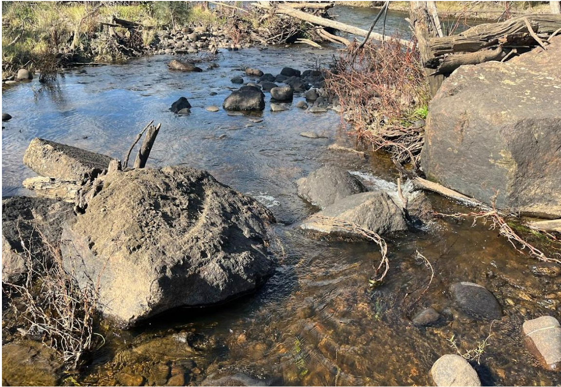
Photo 10: Example of existing weir exhibiting 1:20 grade and avoiding vertical drops greater than 100mm in height and concentrated areas of velocity
